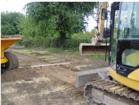
Preparation for concrete raft installation
